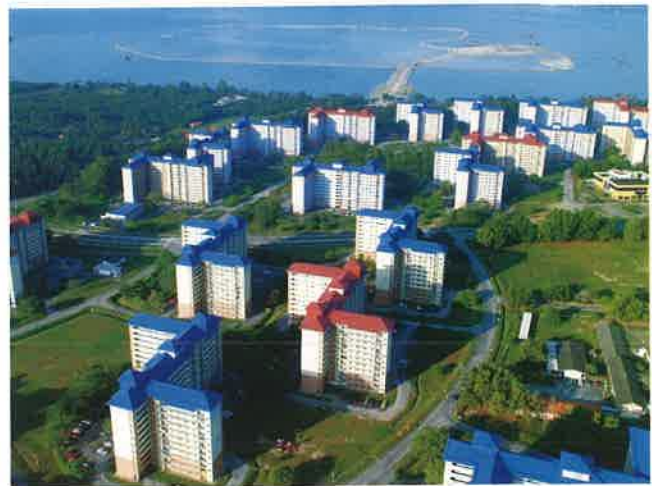
Housing facilities timely maintained by KD MALAYA in order to enhance the living quality of RMN Personnel.
